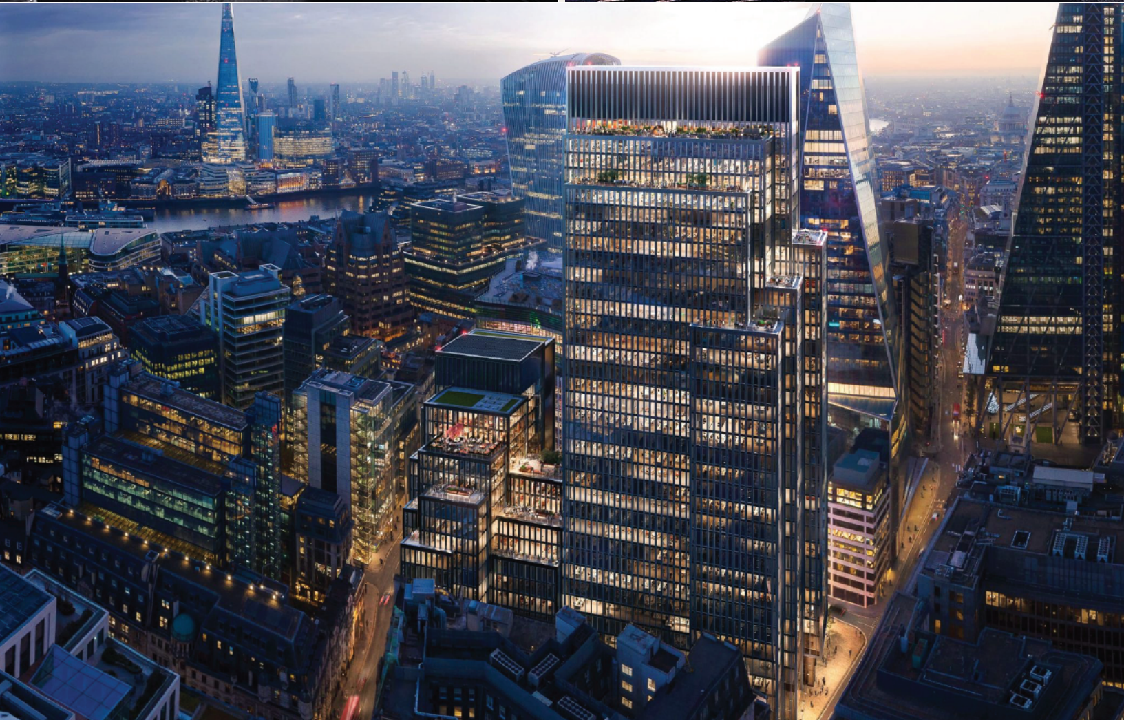
40 Leadenhall Street Screening Room, London
